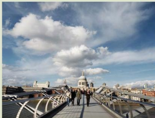
▲ Figure 7 The London Millennium Footbridge.
